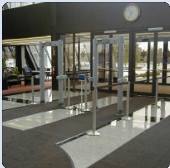
ABOVE: A custom Cyrus Systems installation at a security checkpoint providing dirt, dust and water control and directional benefits.
